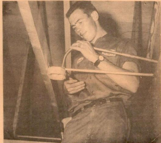
BASE LIBRARY ADDITION -- Buck Ritter of Busby Electric Co. installs conduit which will accommodate the installation of electric wiring at the new addition to the base library. With the added floor space, library officials anticipate greater use of the facility by base personnel. (USAF PHOTO By TSgt. Kapperman)
