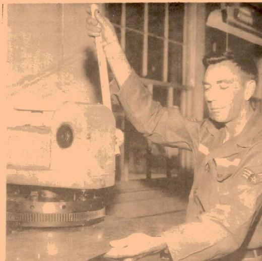
SHEET METAL WORKER -- AIC Walter B. Zisk of the 464th Civil Engineering Squadron punches holes in a piece of sheet metal which will be used to construct a storage bin. The 36-year-old airman's duties consist of making gutters, canopies and heating and air conditioning duct work. The Palmer, Mass., native is also responsible for maintenance of kitchen equipment located at the airmen's dining hall. (USAF PHOTO BY TSgt. Kapperman)
